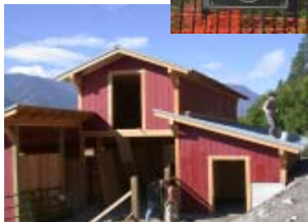
Left: Bear Creek Lumber 1 x 10 STK Red Cedar milled into a channel siding graces this almost finished horse barn in Washington State. Picture by Mark Buck
