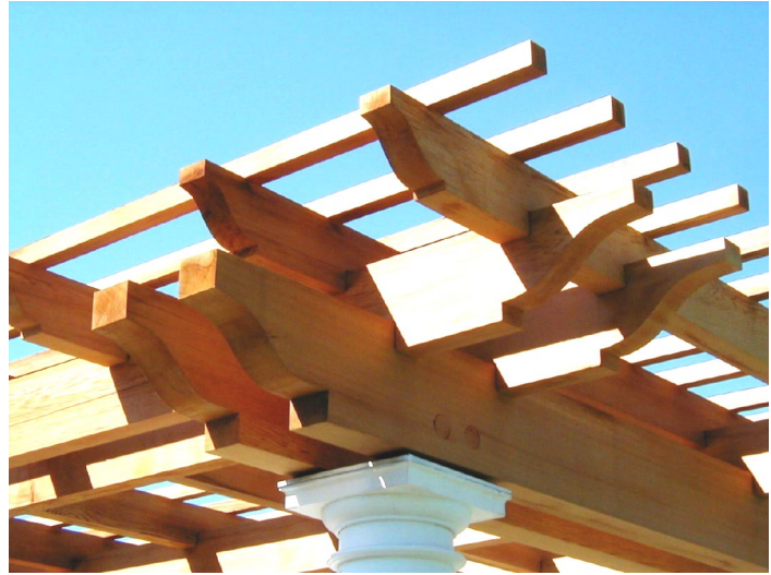
Bear Creek Lumber Clear Western Red Cedar Pergola rafter detail Submitted by Douglas D., Southhampton, NY
