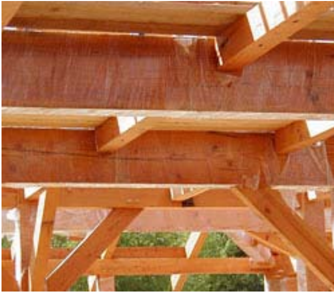
photo of BCL fir beams from www.AlternativeTimberStructures.com Says Porter Broughton, Driggs ID "Great Service, great sales people, great shop people!"
